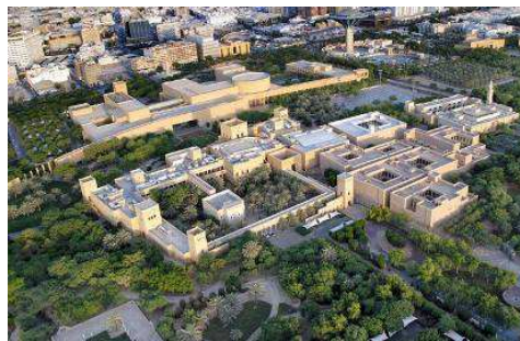
Fig.9: (KAAHC) Traditional and Mud Buildings (Royal Commission for Riyadh City, RCRC)
