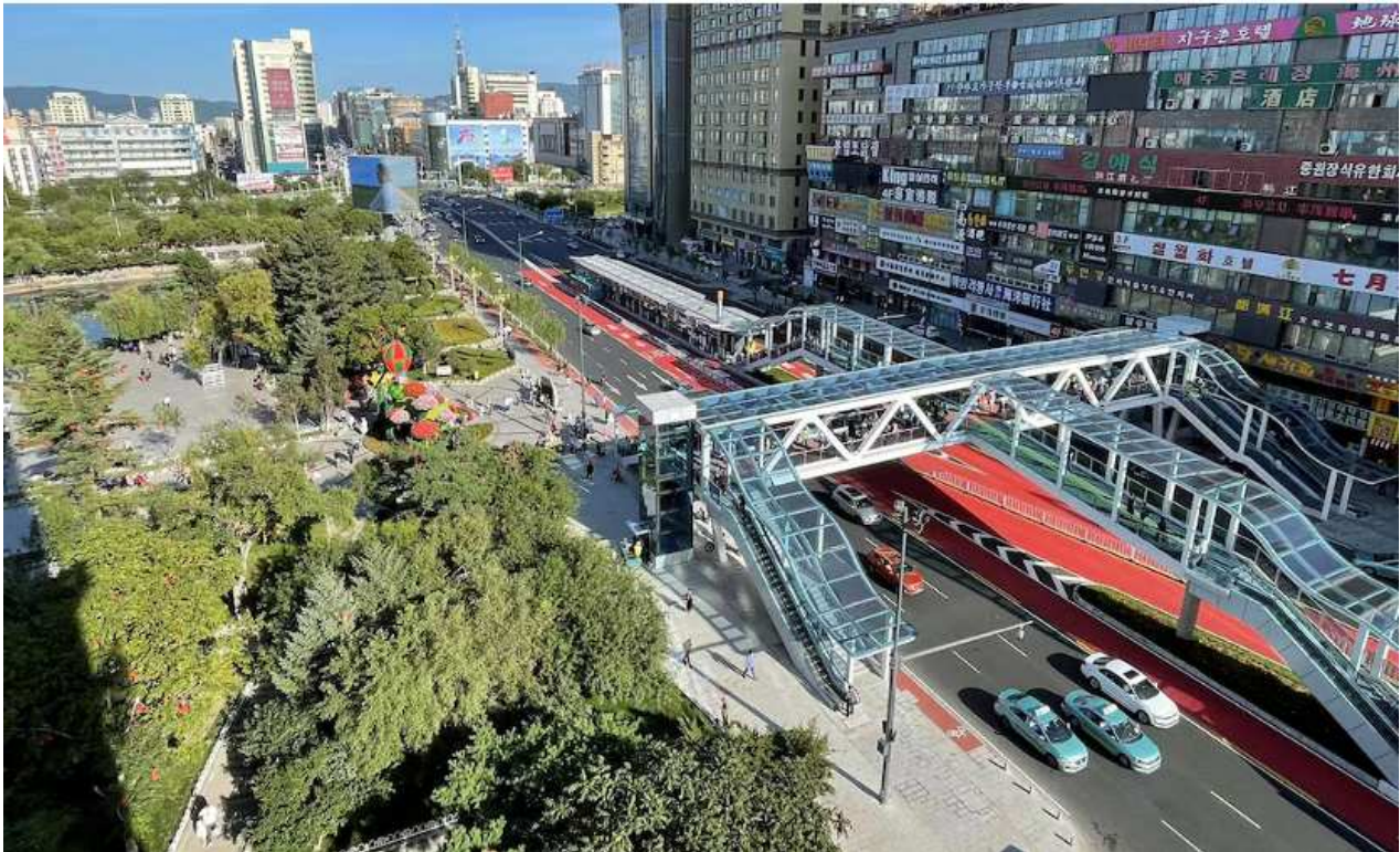
Implemented first phase of the bus-rapid transit with bike paths and sponge city tree planting and road median landscape linking to green parks. Source: Yanji City Government
