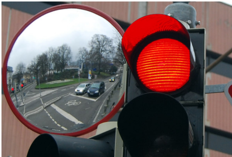
Fig. 7. “Trixi Spiegel” mirror which allows truck drivers to observe cyclist riding parallel (Photo: M. Beim)
