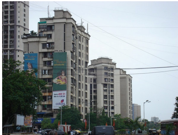
Fig. 5: Typical high-density, high-rise housing
