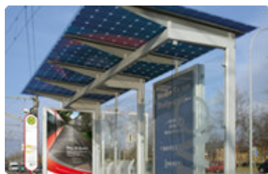
Figure 6: The „Solar Bus Stop in Freiburg, Germany, produces 1.700 kWh/year and its electricity is fed into the grid. (Source: http://www.vag-freiburg.de/wir-ueber-uns/klimaschutz-bei-der-vag.html , 2010)
