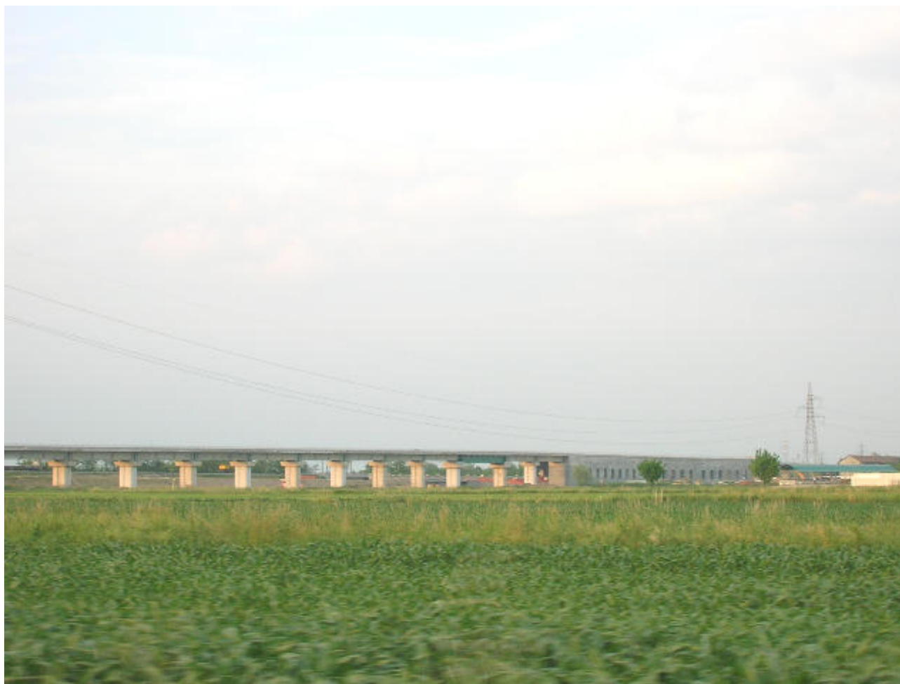
Fig. 1: Work for Milano-Venezia High Speed railway.
