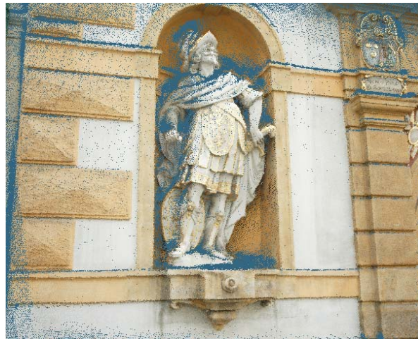
Figure 3: 3D-Model of Province Hall (Landhaus) facade.
