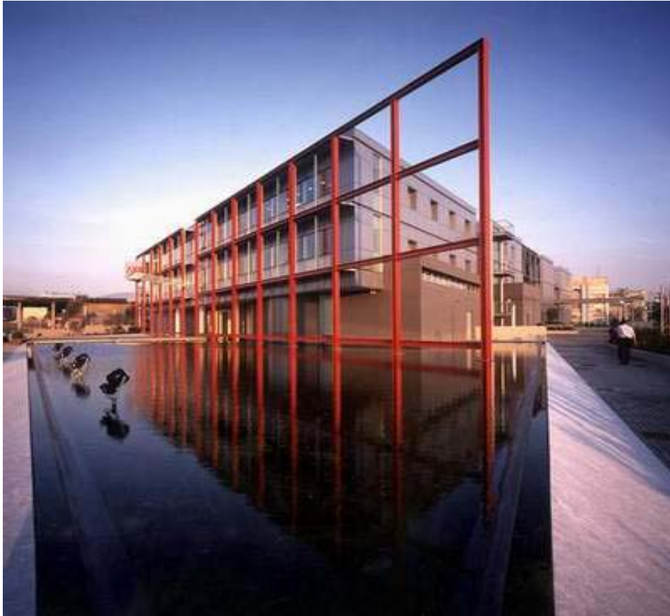
Photo 2: ABB private corporation building in Metamorphossi of Attika
