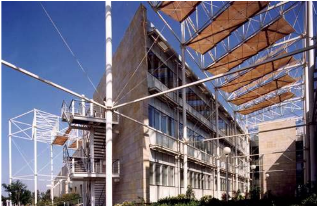
Photo 1: Central Buildings of the Administration of the Public Petrol Corporation "Hellinika Petrelea", in Aspropirgos, Attica.
